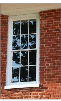
**Lintel**: a horizontal beam over an opening in a masonry wall, which carries the weight of the structure above.
