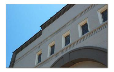
▲ Parapet: low, solid, protective wall or railing along the edge of a roof or balcony. (Also illustrated, *String Course*.)
